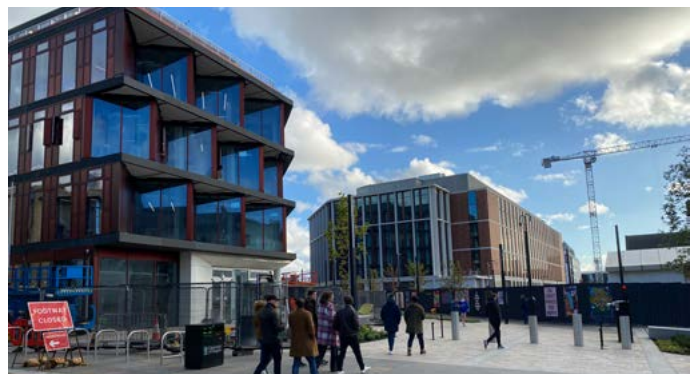
New Campus development opposite
